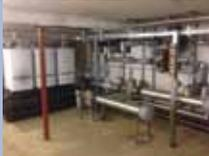
**Hazelbury Primary School** - Design and install two heating plant rooms. Works included asbestos removal and a new Trend control system. Our team were required to work to a very tight schedule, as this contract was completed during term time. Works taking place during breaks due to pupil occupancy.
