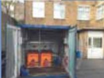
**Lea Bridge Road Temporary Residency** - We provided heating and hot water to 56 flats with our own gas-fired 120Kw containerised boiler plant, to enable works to replace faulty boilers. Install and modify existing kitchen, bathroom and roof extract fans, complete with remote controls.
